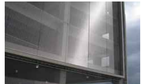
Thanks to its transparency, stainless-steel mesh allows good circulation of air.
