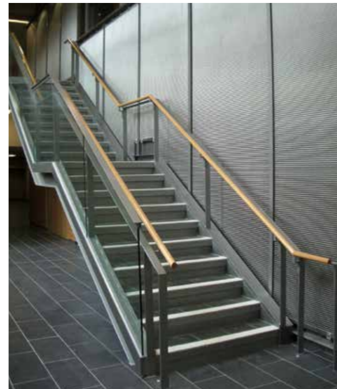
Staircase wall covering. Lamton Hall, Guelph, Ontario, Canada.
