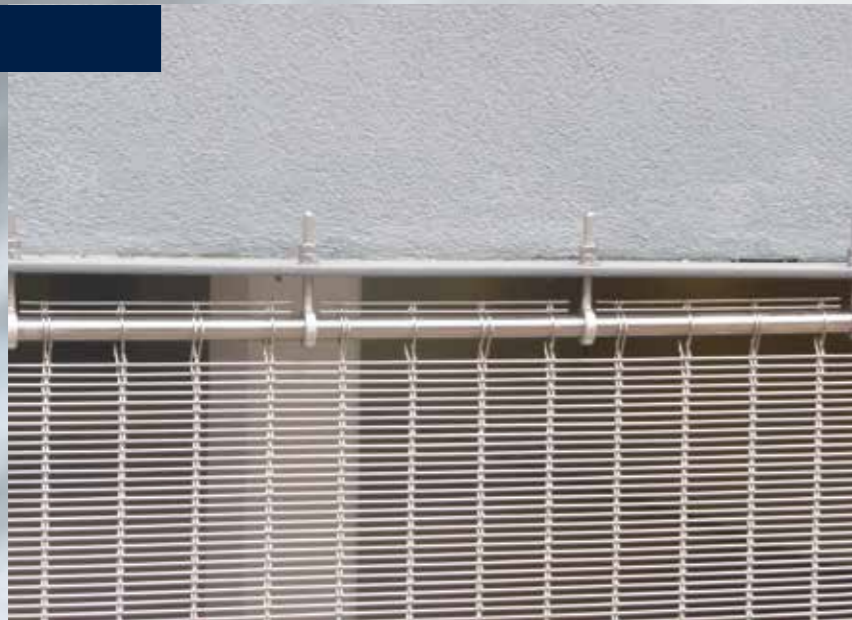
Top mounting: round bar with eyebolts.
