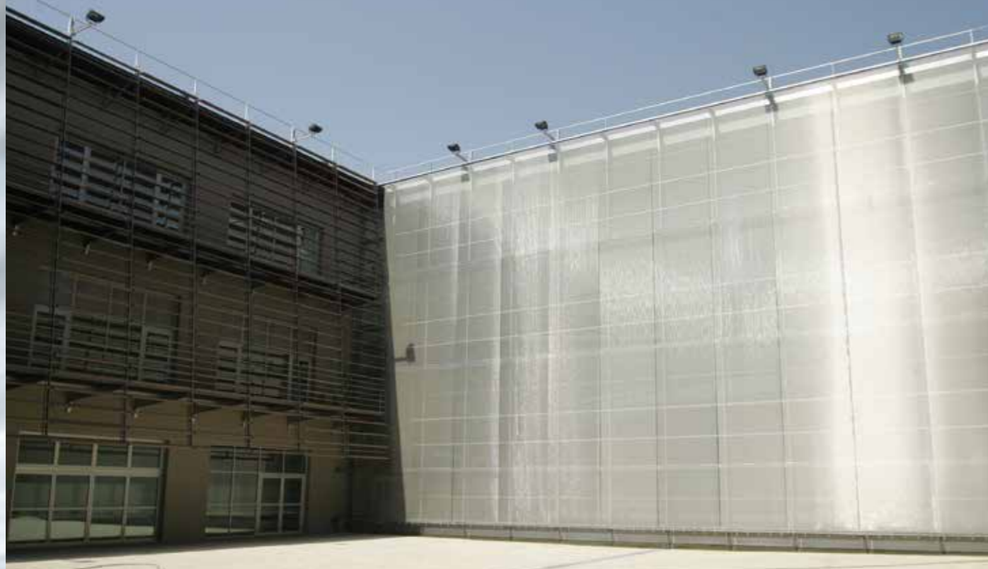
Privacy during the day. EGLA-TWIN mesh façade, Benaki Museum, Athens, Greece.
