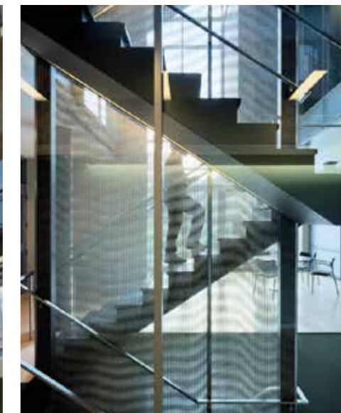
Stairwell cladding using two layers of architectural mesh to create the moiré effect. McGill University, Montreal, Canada.
