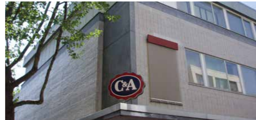
A semi-transparent stainless-steel mesh encloses the existing building and ensures natural lighting. C&A Eco Store, Mainz, Germany.
