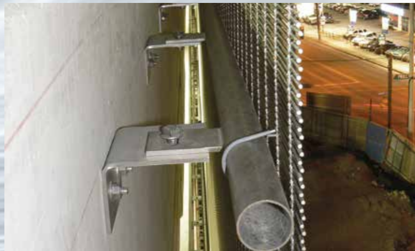
Intermediate mounting: round tube and wire connectors.
