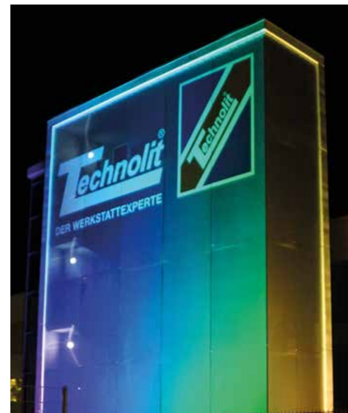
Mesh illumination and painted lettering. Technolit, Großenlüder, Germany.
