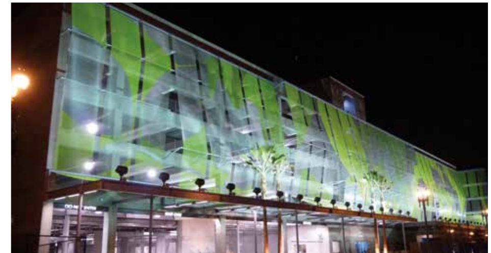
Partially painted mesh elements. Los Angeles Police Department Car Park, USA.
