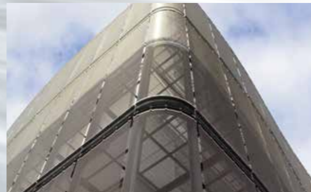
Corner segment with pre-rounded elements: Holland Park School, London, Great Britain.
