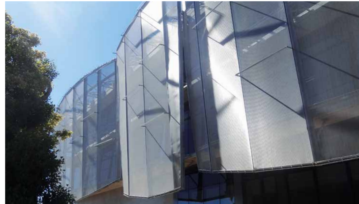
With puristic aesthetics, the shimmering metallic effect of the stainless-steel mesh in sunlight brings out the overall architectural concept.
