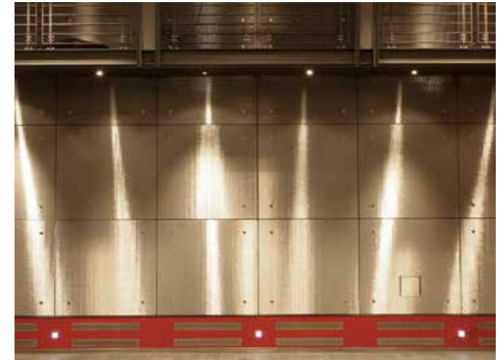
Architectural mesh makes the walls of the proscenium at Luxembourg's Théâtre Municipal shine.
