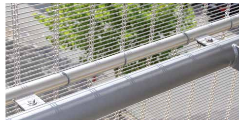
Intermediate mounting: round tube and wire connectors.
