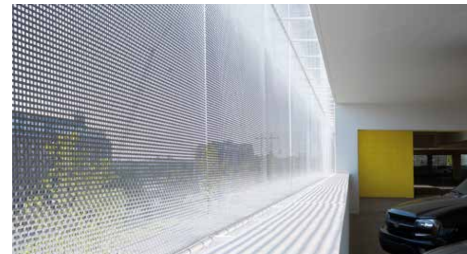
Sun protection with a good view from inside. Multi-storey car park, Chesapeake, Oklahoma, USA.
