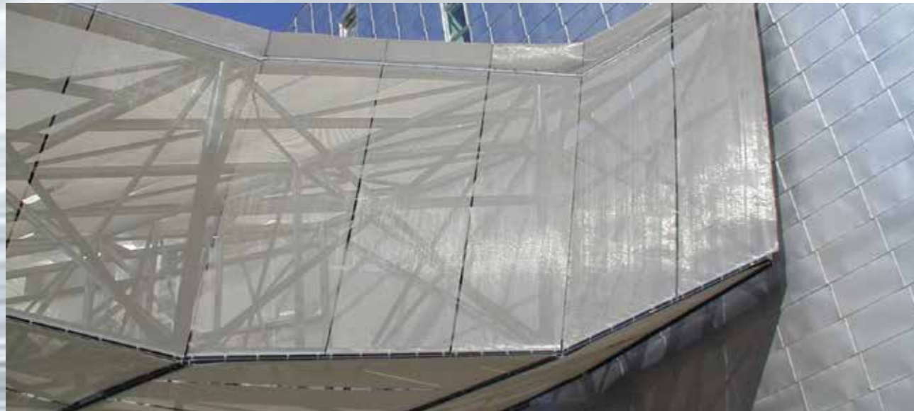
Three-dimensional canopy with individually tensioned elements: Malaga Exhibition Centre, Spain.
