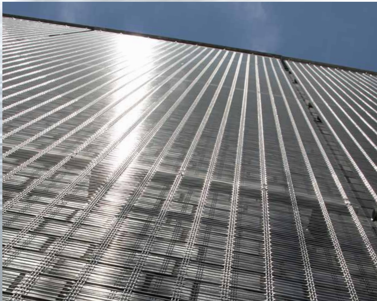
Architectural mesh can be tensioned vertically over several storeys. Load-bearing substructures are only required on the upper and lower face.
