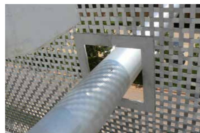
Cut-outs in mesh elements.
