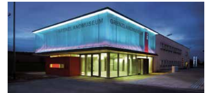
Night-time view with backlit wire mesh.
