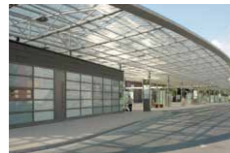
Wire mesh as sun protection. Herne Bus Station, Germany.
