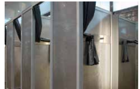
Changing room featuring architectural mesh. Mode-Boutique, London, Great Britain.
