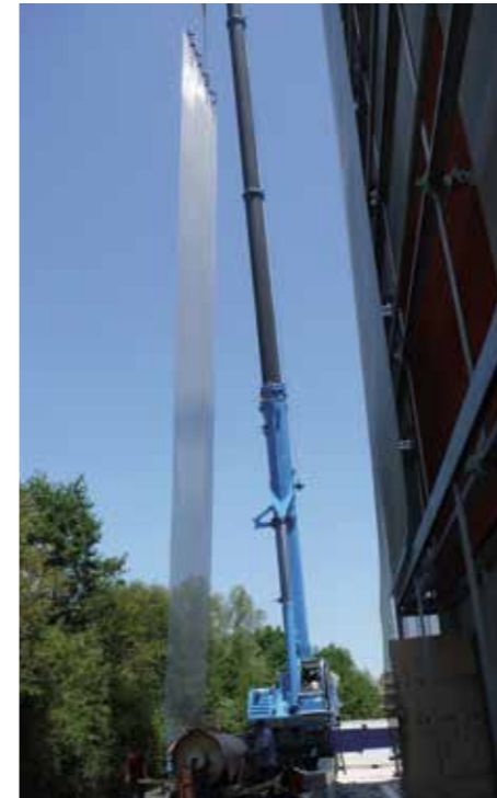
Large mesh elements are quick and easy to assemble. Once assembled, HAVER Architectural Mesh requires little to no maintenance.
