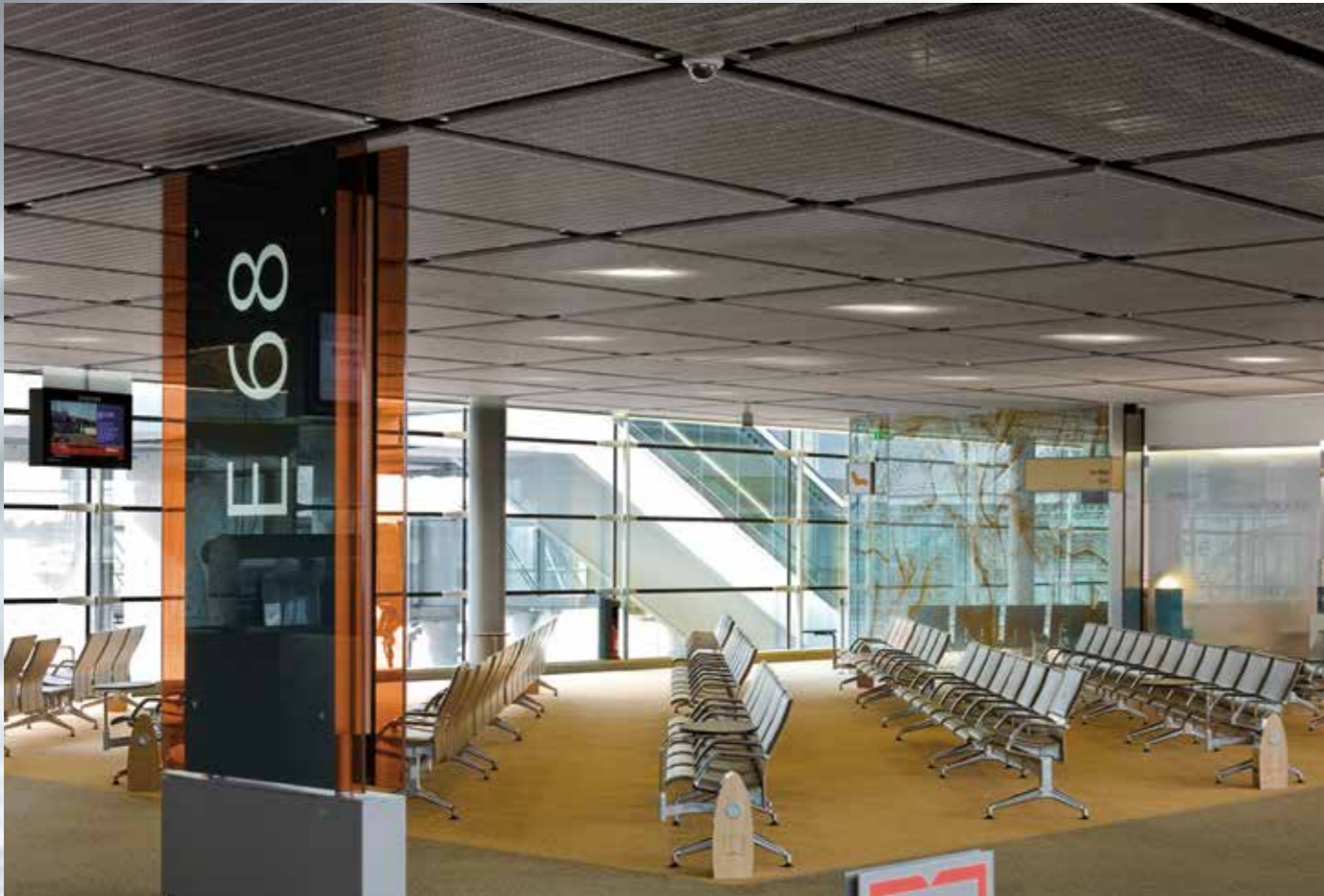
Architectural wire mesh guarantees the optimum operation of ventilation or sprinkler systems Terminal S3, Roissy Charles de Gaulle Airport, Paris, France.
