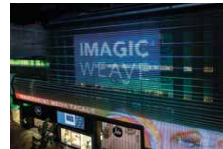
18 different resolution ranges on one façade. Júlia Center, Andorra la Vella, Andorra.
