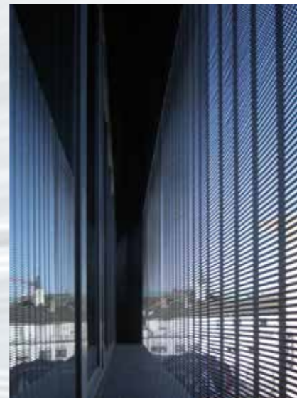
The open geometry of the architectural wire mesh preserves the view on the outside world.
