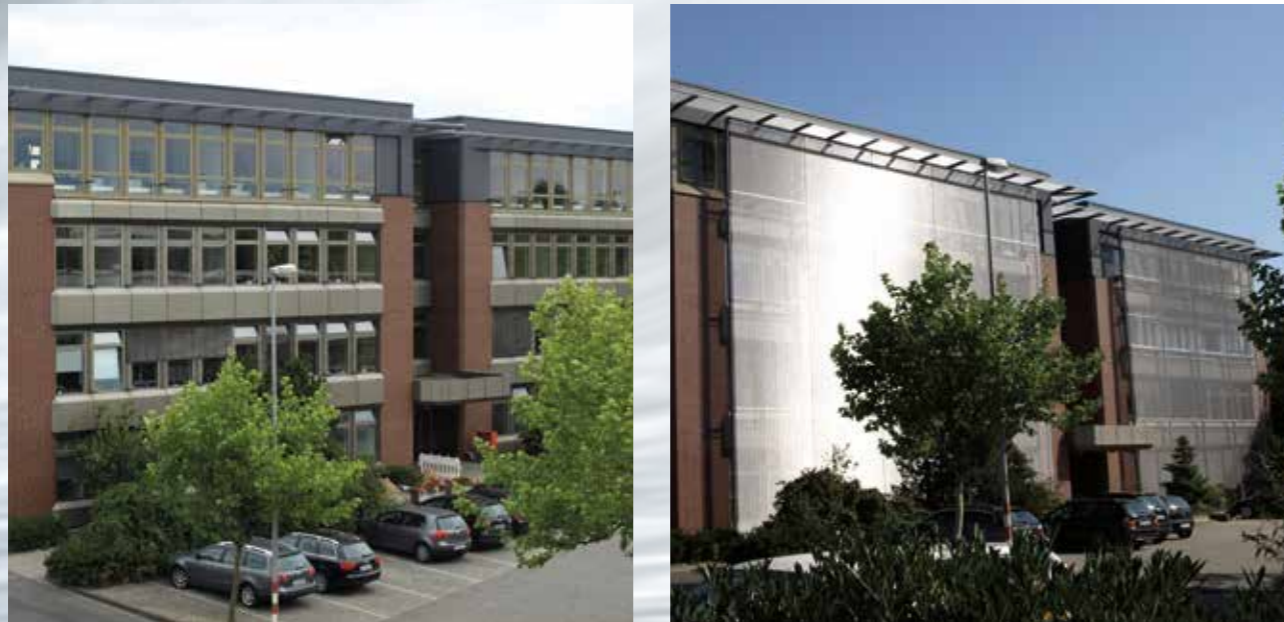
DOGLA-TRIO blends the newly added floor with the existing structure. Haver & Boecker, Oelde, Germany.
