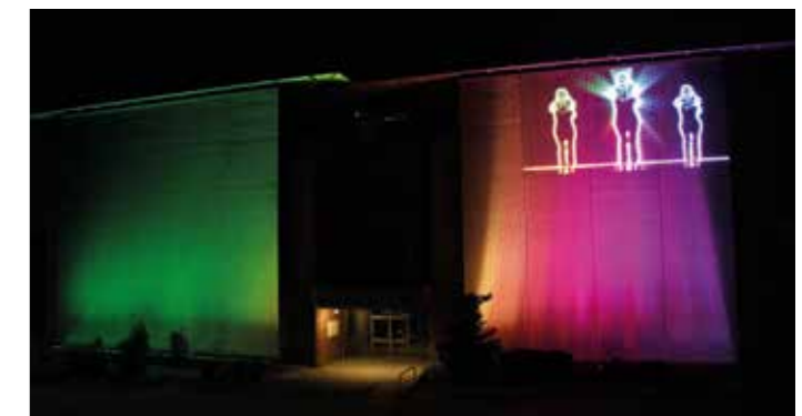
Mesh illumination. Haver & Boecker office building, Oelde, Germany.
