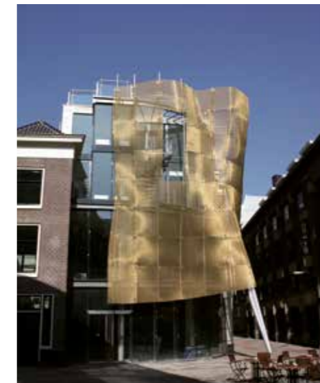
Freely formed stainless-steel mesh. De Baljurk, Kettingstraat, The Hague, Netherlands.
