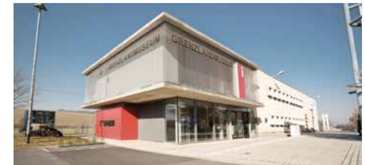
EGLA-TWIN wire mesh façade during the day. Eichsfeld Borderland Museum, Teistungen, Germany.
