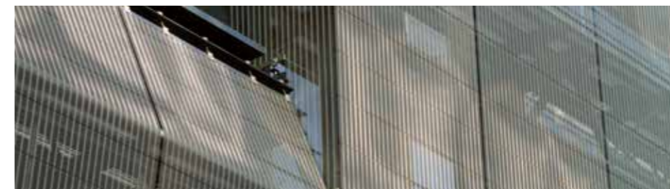
Multidimensional façade with mesh elements deflected by 19°. Júlia Center, Andorra la Vella, Andorra.
