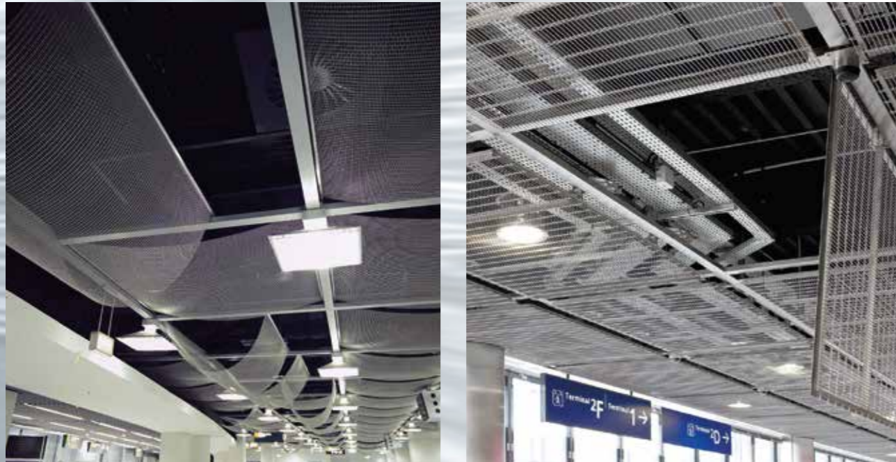
Adjustable mounting system for ceilings with sag.
